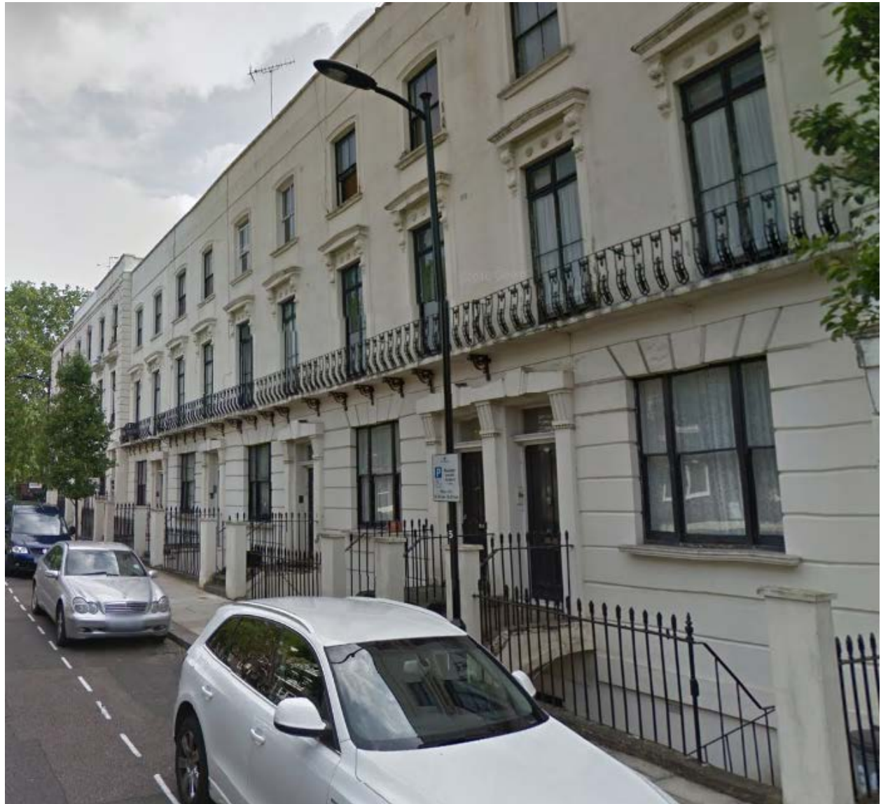
Front elevation of Nos.32-34 Blomfield Villas.
